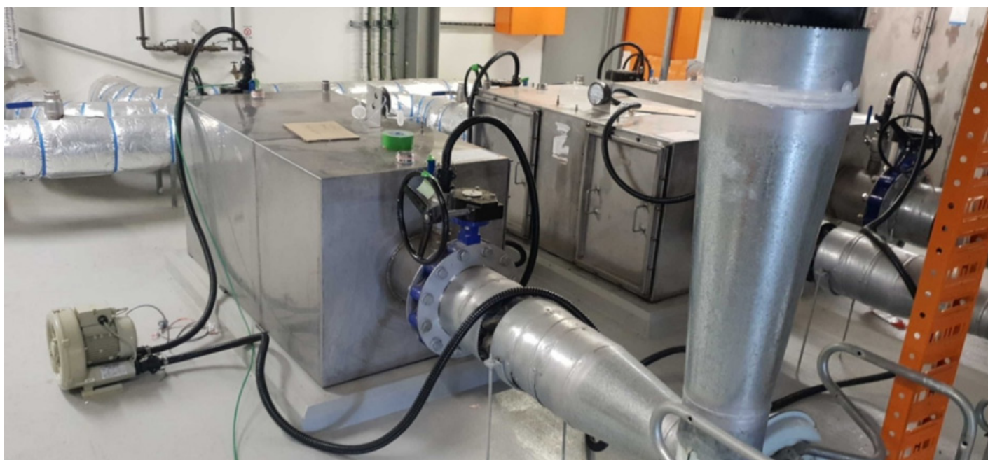
Figure 4 - A typical HEPA Housing and Side-Channel Blower set up in actual in-situ image.
